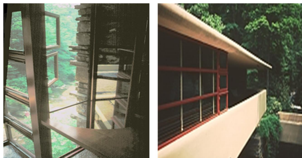
Fig. 3. Installing all windows and removing the corners of the room
